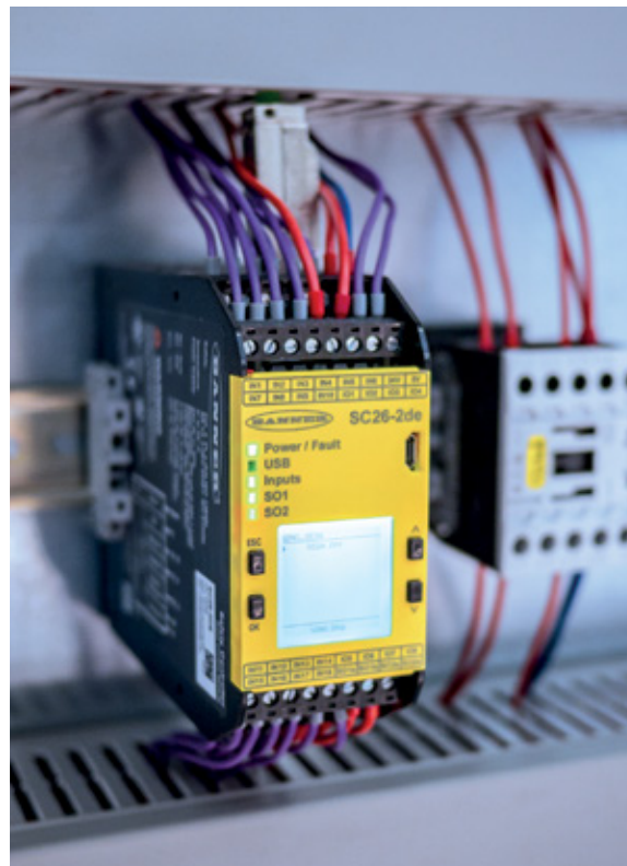
Banner's SC26-2 safety controller controls the safety functions of the machine
